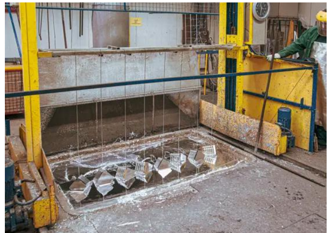
Hot-dip galvanizing plant (2003)
